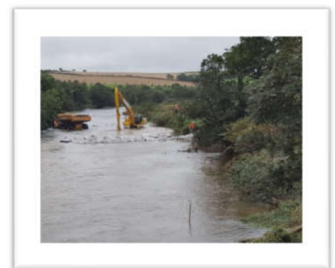
Figure 1 Dredging works - Bandon River 2016
