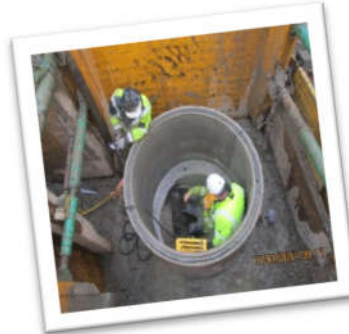
New man hole installation
