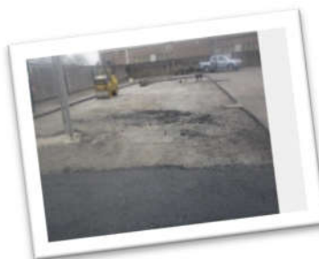
Resurfacing Work to completed area after drainage works
